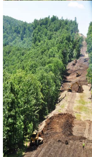
Pipeline construction in the Marcellus Shale.
