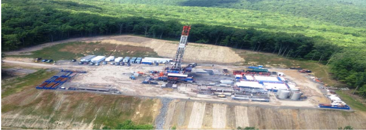
Drilling operation in the Marcellus Shale.
