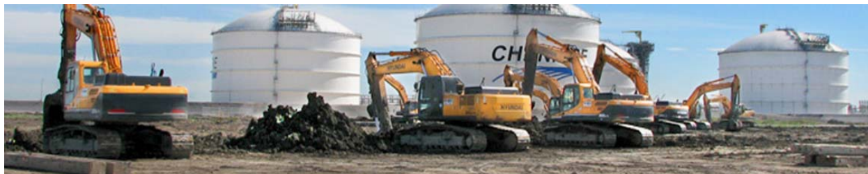
Cheniere LNG facilities construction.
